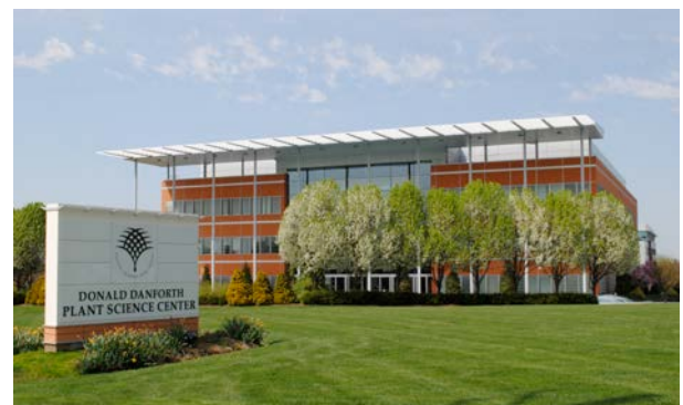
The Donald Danforth Plant Science Center in St. Louis, MO.
